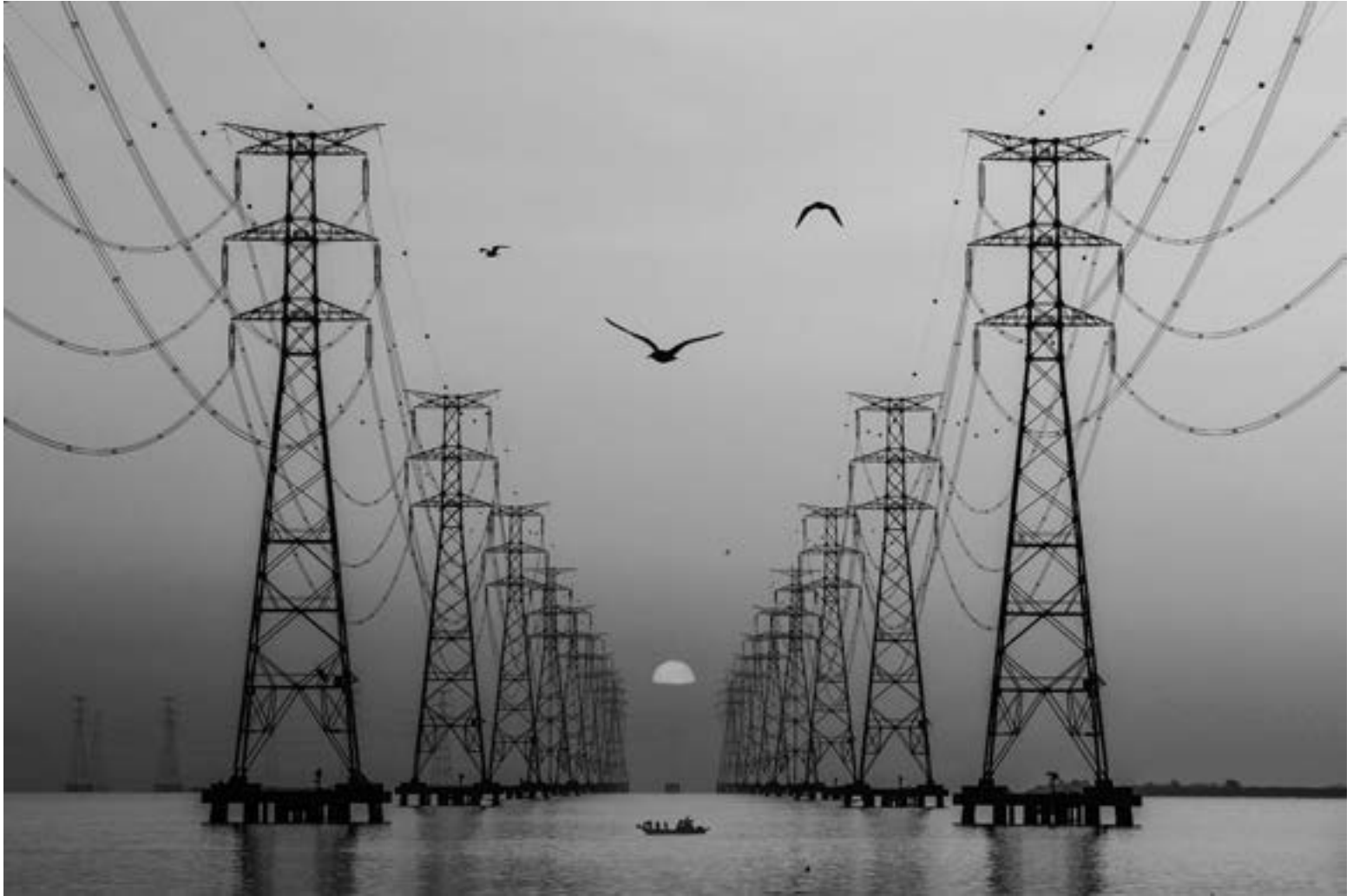
Shin Woo Ryu, South Korea, Transmission Line
